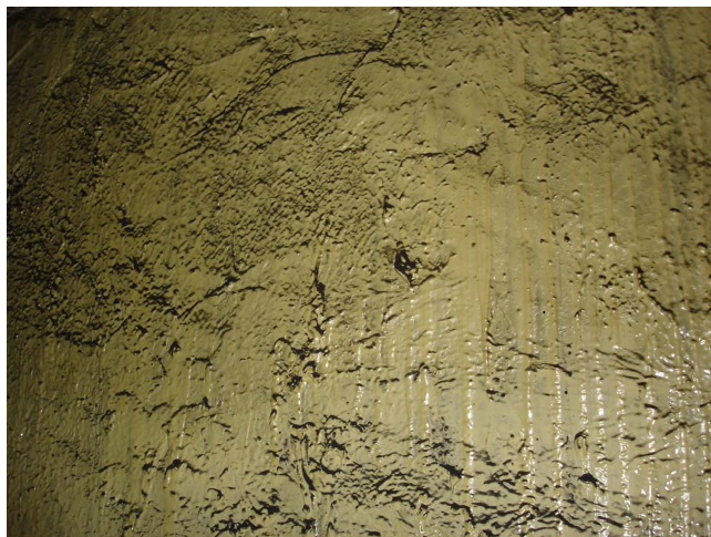
Figure 7. Photograph of modified PUE applied to coal mine. [Color figure can be viewed in the online issue, which is available at wileyonlinelibrary.com .]
